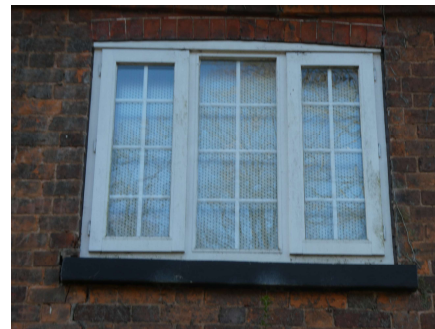
View of typical timber window installation.
