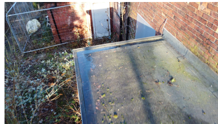
View of blistering to the mineral felt roof covering.
