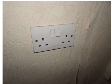
View of dated socket face plate to the ground floor areas.
