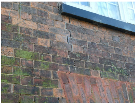
View of stepped cracking to front elevation between the dining room and bedroom window.
