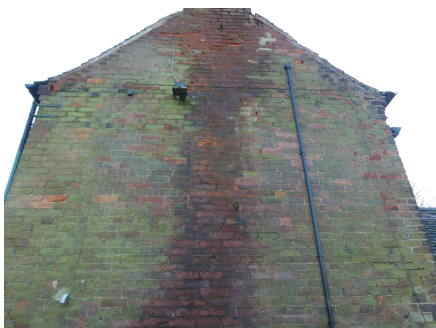
View of damp staining to the right hand side elevation brickwork.
