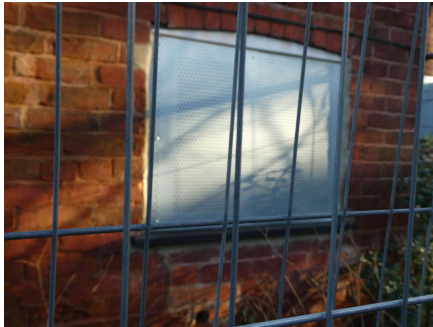
View of typical metal sheeting installed to the face of the ground floor windows.
