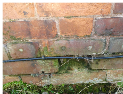
View of chemical damp proof course to the low level masonry brickwork.
