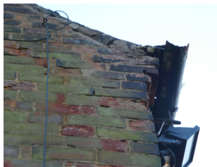
View of corroded and part missing cast iron gutter.
