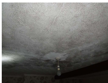
View of cracking to the first floor bedroom ceiling.
