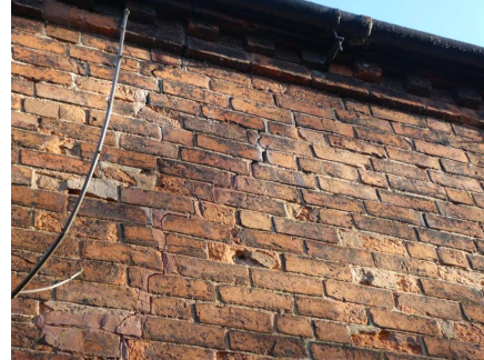
View of the cracking to the rear elevation external brickwork at high level.
