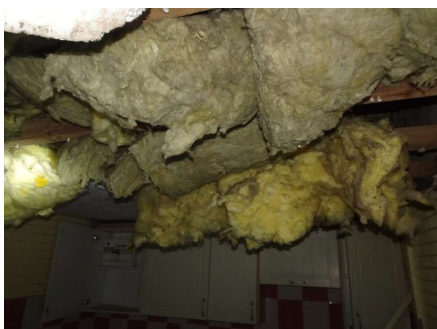
View of the collapsed kitchen ceiling.
