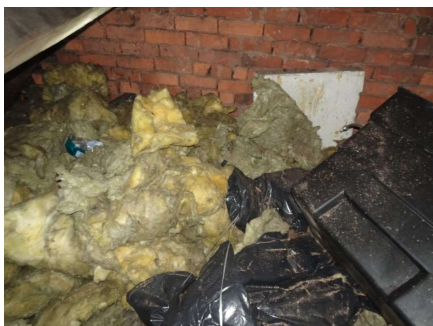
View of damaged insulation.
