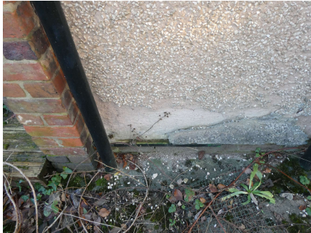
View of the cracked and part missing pebbledash rendered coating.
