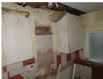
View of the damaged plasterwork to the kitchen area.
