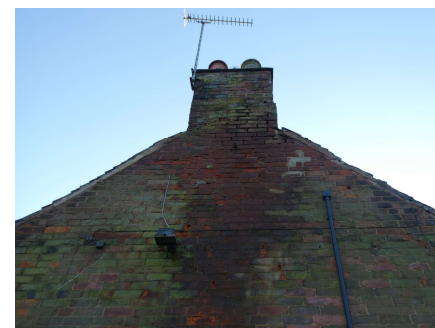
Further view of damp staining to the right hand side elevation brickwork at high level.
