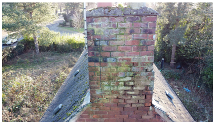
View of degraded and part missing mortar pointing to the chimney stack.
