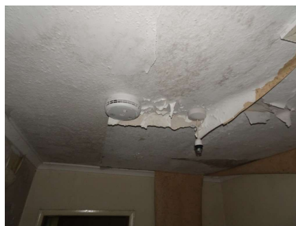
View of delaminated decorative ceiling covering to the landing area.
