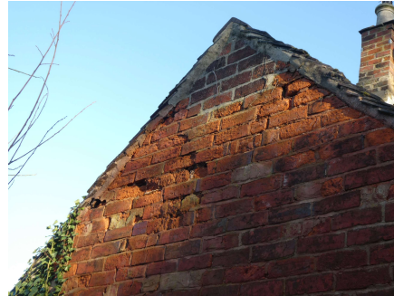
View of spalled and cracked brickwork and degraded mortar pointing.
