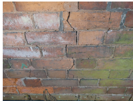
View of the stepped cracking below the living room window.
