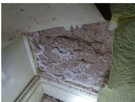
View of cracked, crumbling, and damaged plasterwork to the first floor bedroom.
